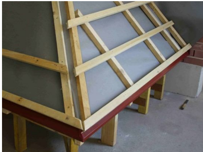
Breathable membrane – GROIN OF ROOF
